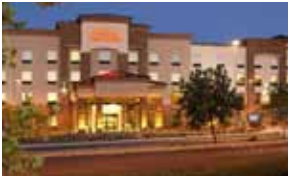
A.R. Mays Construction
