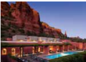
Phil Morris Construction
